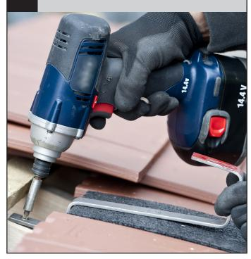
Place the tiles over the HookStop<sup>™</sup> to make weatherproof.
