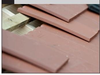
Replace the tile directly under where the REDtip roof hook is to be fitted with a HookStop<sup>™</sup> and fit directly onto the roof batten with the appropriate fixing.
